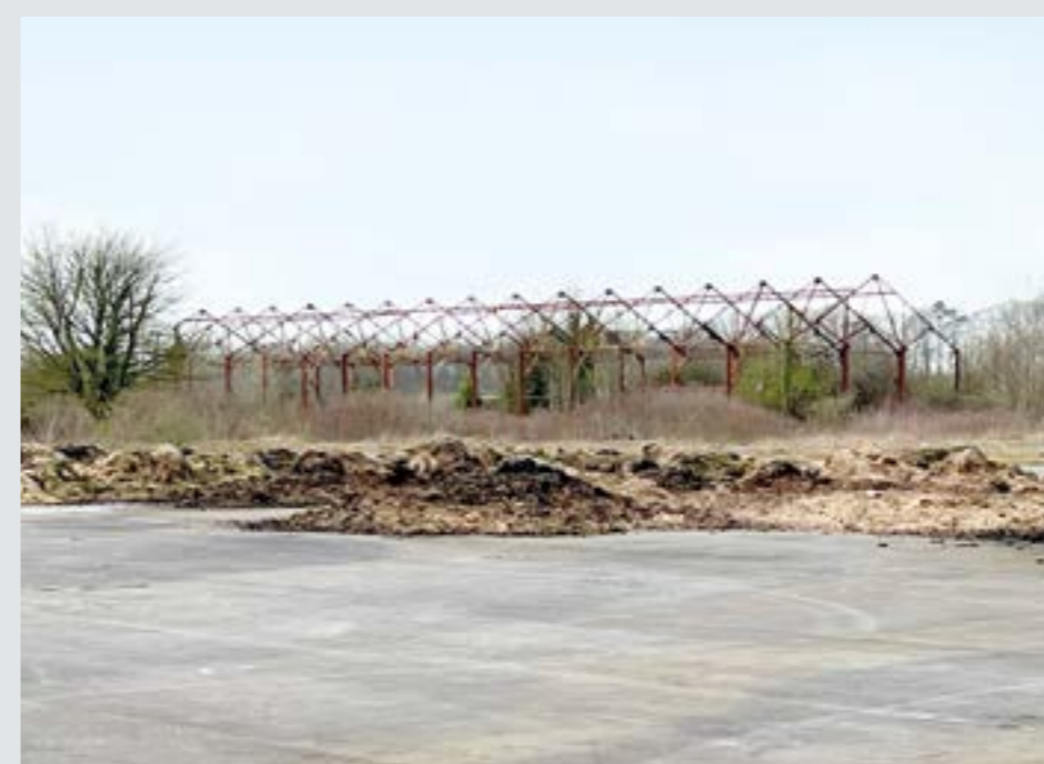
Bushfield Camp's parade ground with the steel frame of the gymnasium building behind it.
