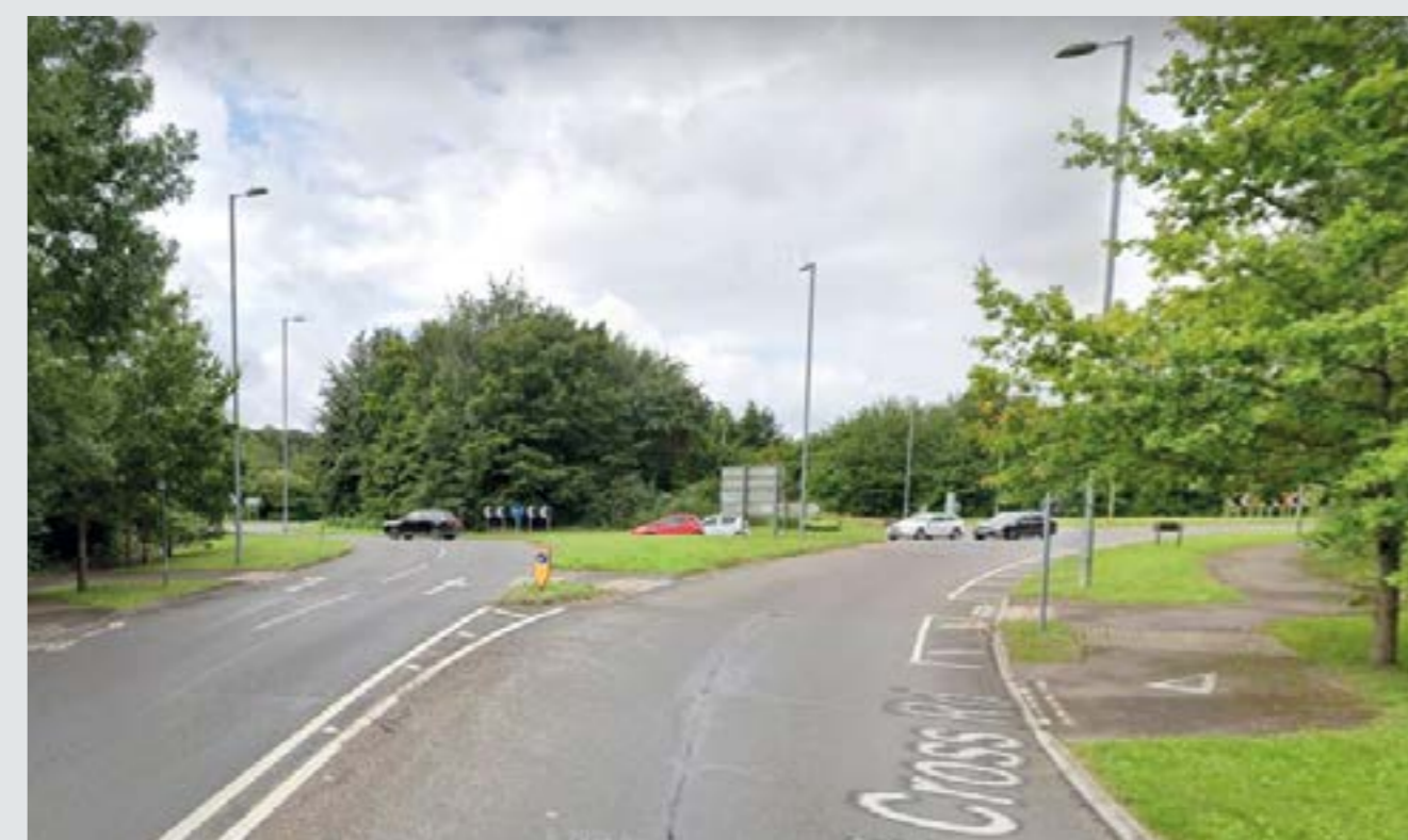
Difficult pedestrian/cycle environment at St Cross Roundabout.
